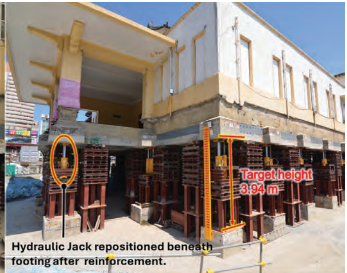
Figure 5: The second phase of jacking.
