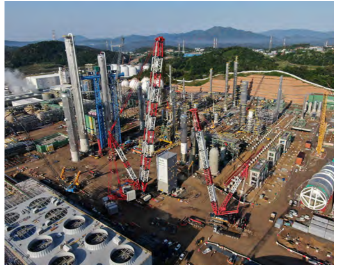
Denzai's LR12500 and LR11350 crawler cranes lifting a 902-t cold box on the S-Oil Shaheen Project.
