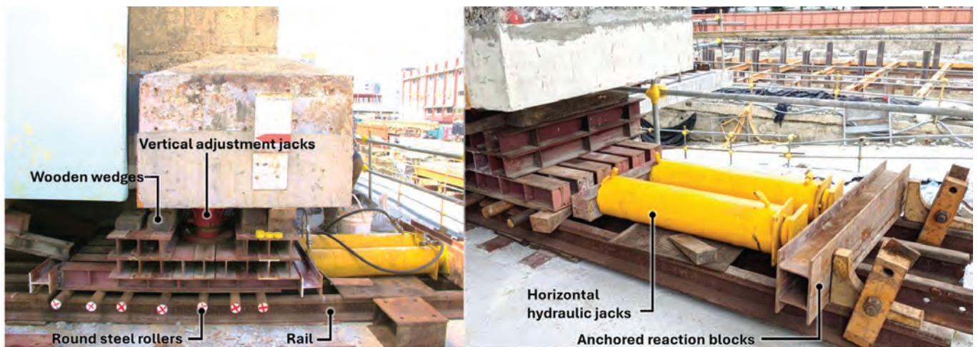
Figure 8: Moving assemblies and pushing devices.
