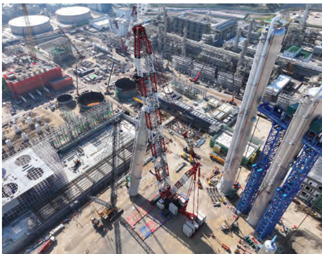
Denzai's crawler cranes lifting a 973-t component.
